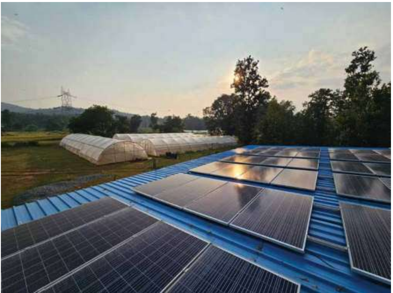
Solar micro-grid for irrigation at the farms
