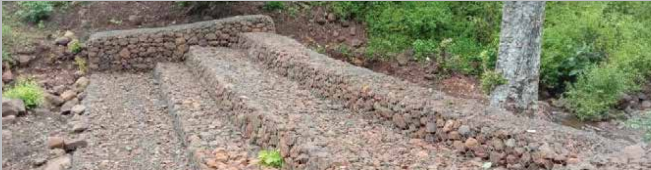
Large scale land husbandry to check soil erosion: This work was undertaken in 11,762 ha of area. The aim was to treat the erosion-prone uplands by ways of land levelling, bunding, contouring and construction of staggered trenches. Such interventions checked water run-off, thereby preventing soil erosion. These interventions supported 25,193 households.
