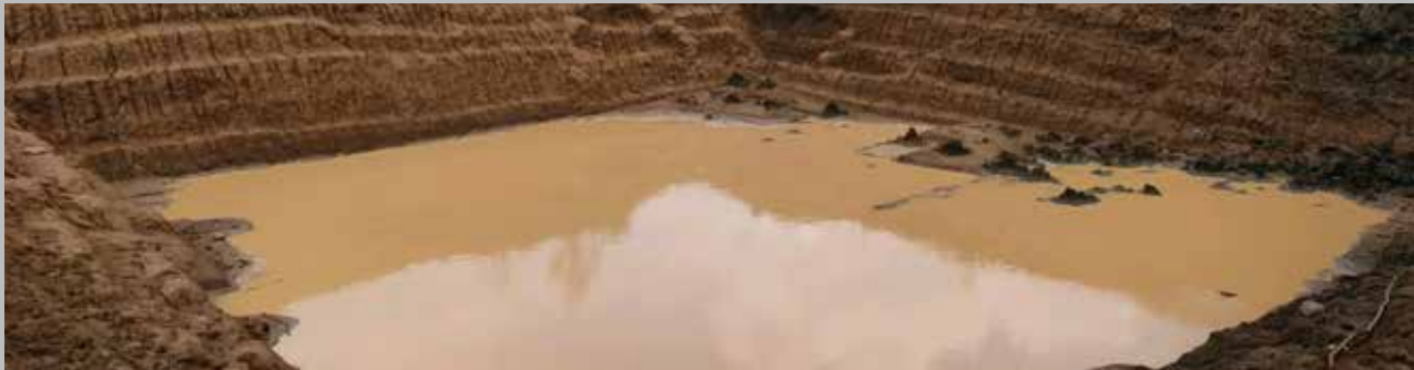
Creation of decentralized water harvesting tanks (WHT): This helped in storing excess water from precipitation, allowed water recharge, improved the hydrology of the area and reduced the risk of crop failure, as the farmers used the stored water to provide emergency irrigation to cereal crops during drought spells. Over 25,604 irrigation infrastructure projects were undertaken to support about 55,645 farmers, in order to save their crops.
