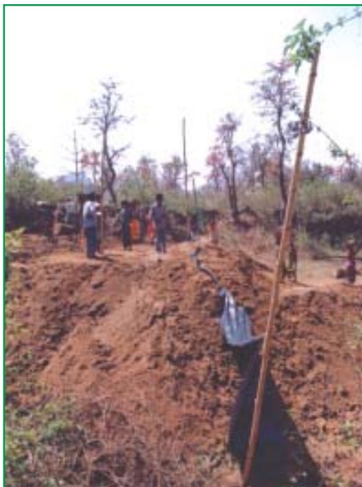
Providing water line for agriculture land.
