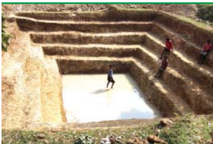
Excavation of tanks with 1:1 slope.
