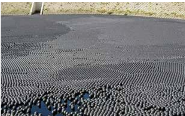
Photo 6: Example of shade balls (Source: 'Shade Balls' Roll their Way into the Spotlight | Energy Vulture)
