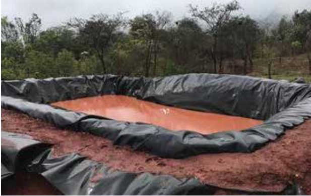
Photo 4: Example of a lined pond in Kitui, Kenya (Source: MetaMeta).
