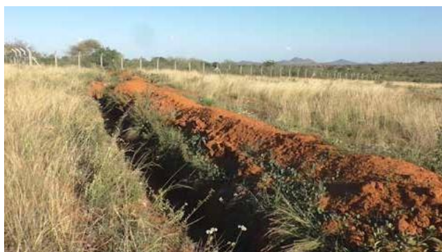
Figure 5: trenches ensure water can slowly infiltrate and thereby prolong duration with higher soil moisture
