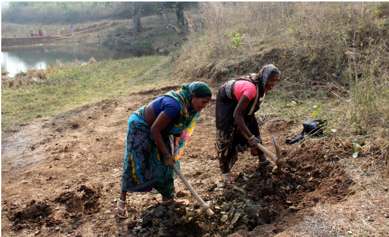
Women sharing labour to terrace the slopes for checking soil erosion, Deosar, MP
